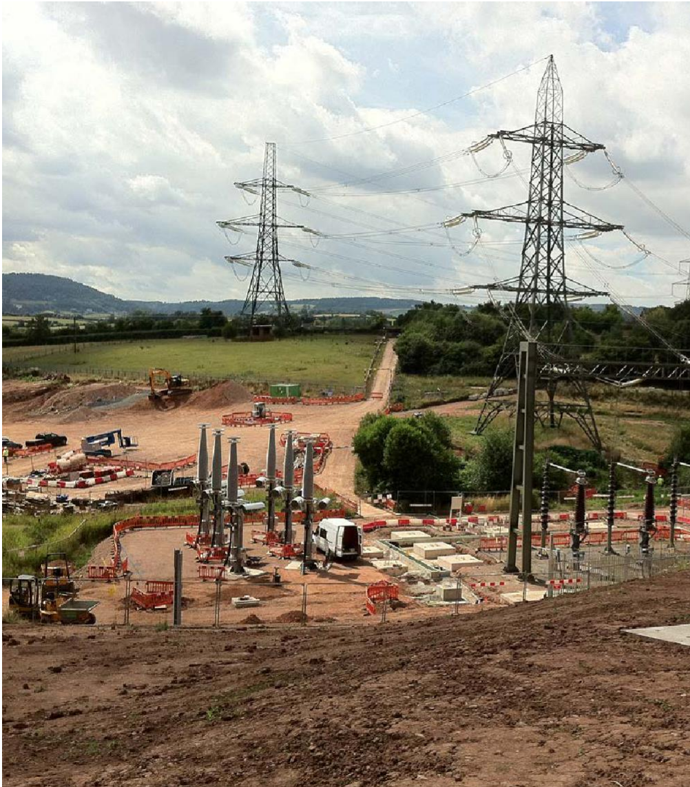
The undergrounding of electricity cables at Ross-on-Wye
